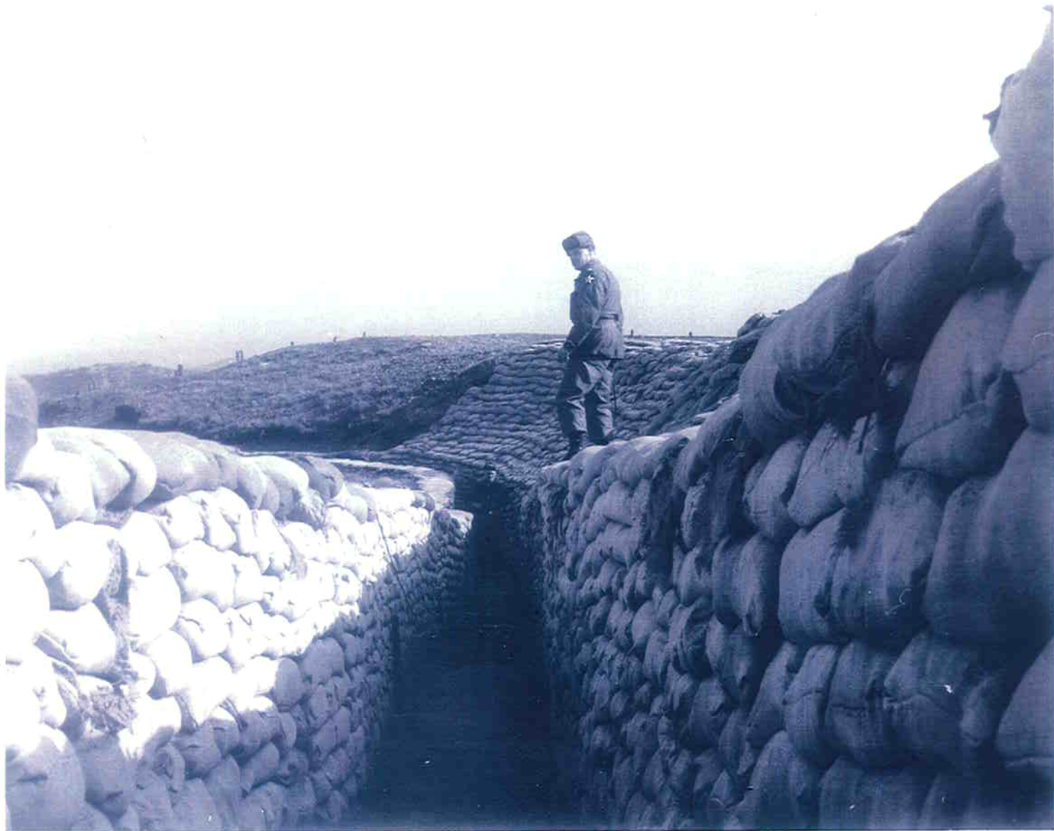
(Korea Demilitarized Zone (DMZ) 1966)... 1 LT Martin J. O'Grady, B/2/23 IN (M), checks the sandbags reinforcing a communications trench at a Guard Post (GP) in the Demilitarized Zone (DMZ). The sandbags would keep the trench from collapsing in the event of bombardment and provide protection from small arms fire. Various fighting positions were located along the trenches that ringed the position.
